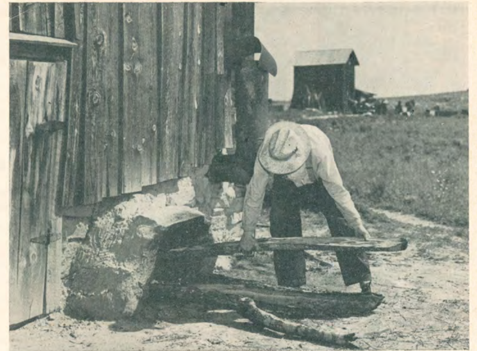
The fire is built from the outside and the resultant heat is carried through the barn in long, metal flues. In this method the leaf is heat cured without smoke.
