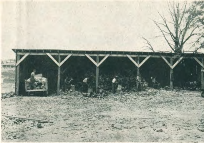
When first brought in from the fields the briar burls are stored in huge sheds (left) until such time as they are cleaned and sent to a large room (right) where they are first cut into huge uniform slabs by these circular 32 inch power saws.
