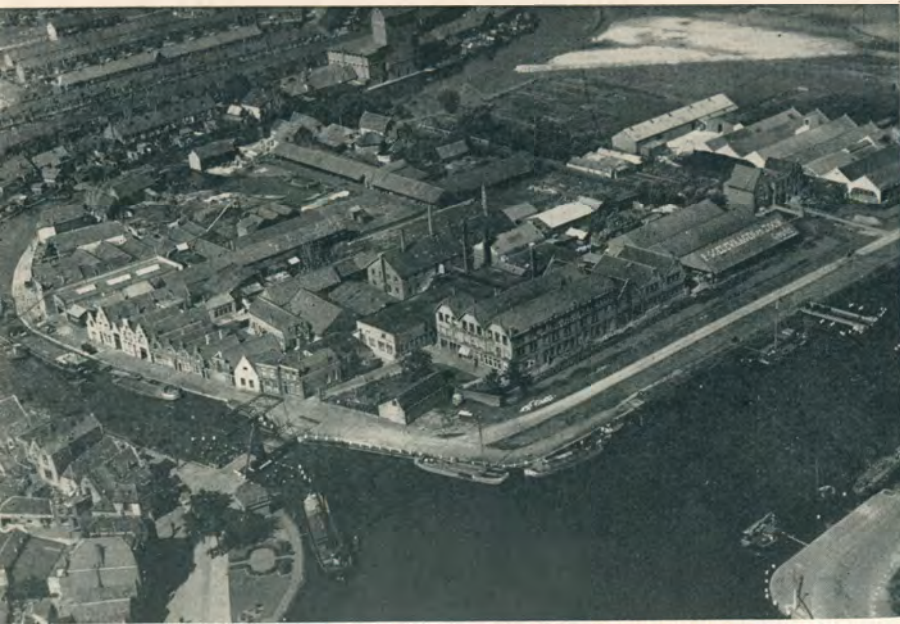
Left, air view of the factory buildings at Gouda, Holland. Bottom, display room which shows many types of pipes made.
