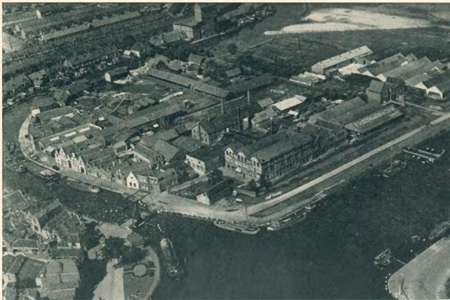
Left, air view of the factory buildings at Gouda, Holland. Bottom, display room which shows many types of pipes made.
