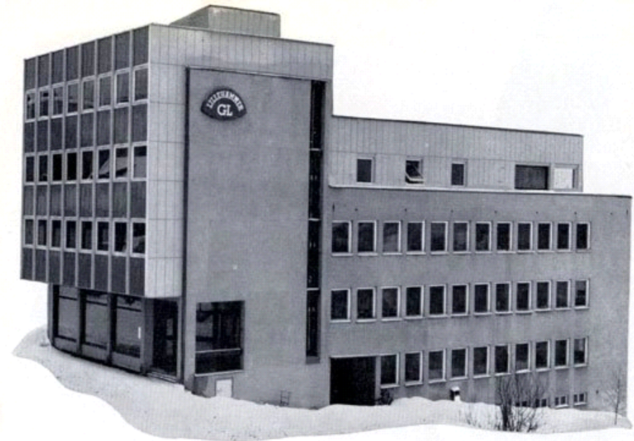
The factory building which after the latest extension was completed in 1965.
